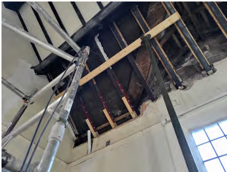
Figure 8: Timber Repair Works - Remedial Works to Main Hall.
