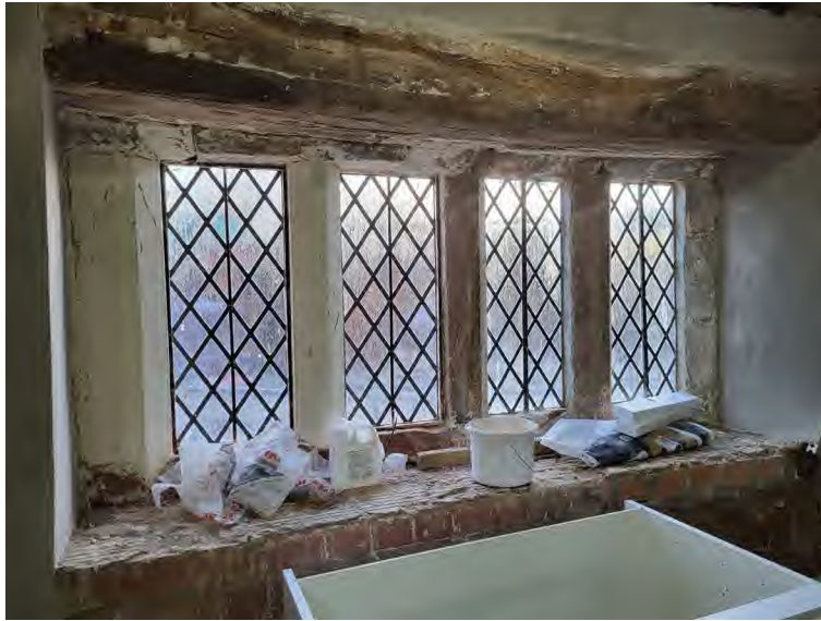
Figure 10: Existing Kitchen - Mullions to be Limewashed.
