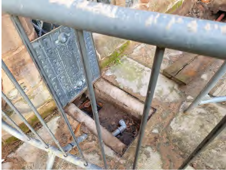
Figure 13: Drainage Works - Waste from Kitchen Reviewed.
