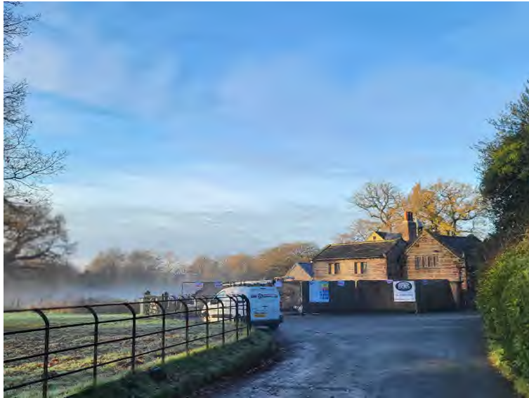
Figure 1: General View of Works.
