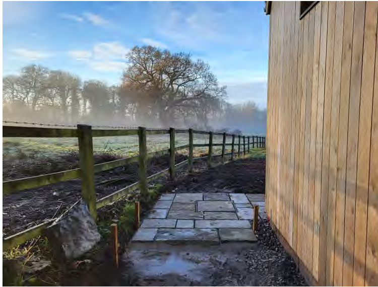
Figure 4: Landscaping - Stone Paving and Manhole Cover.
