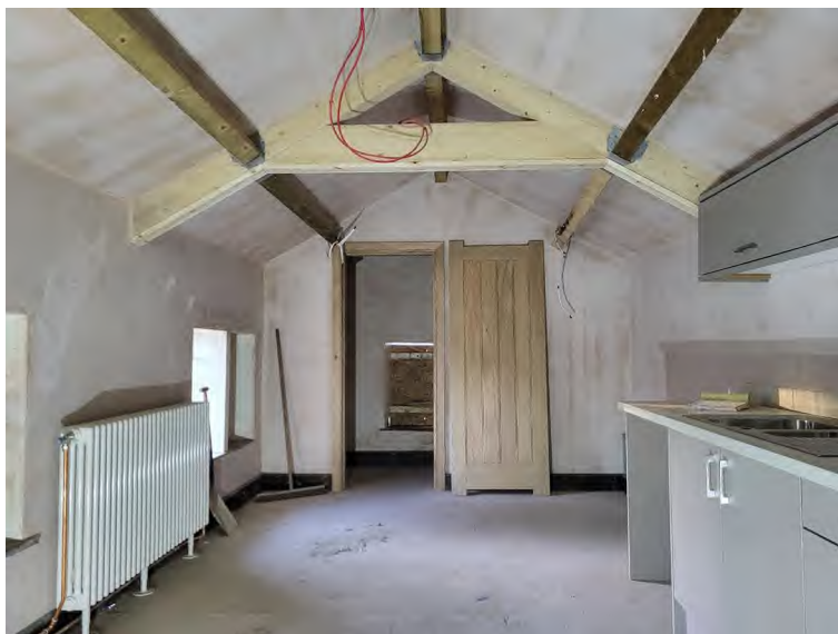
Figure 3: General View of First Floor.
