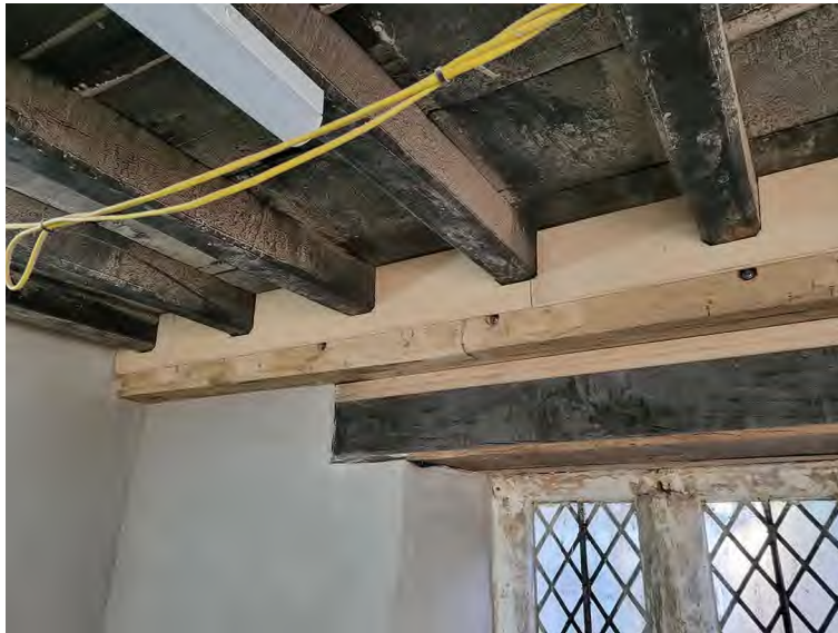
Figure 11: Existing Kitchen - Joinery to be Stained Dark.
