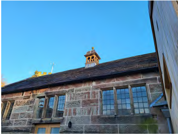
Figure 7: Completed Works to Bellcote.
