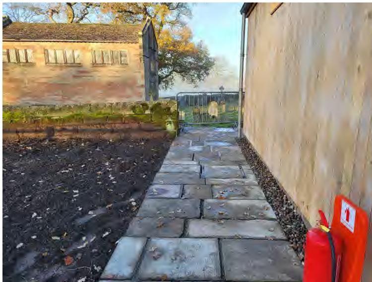
Figure 5: Landscaping - Stone Paving and Manhole Cover.
