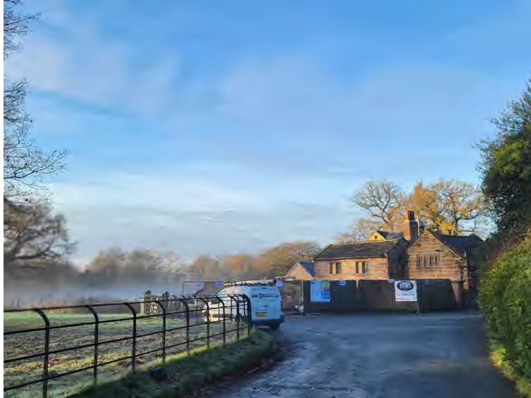
Figure 1: General View of Works.
