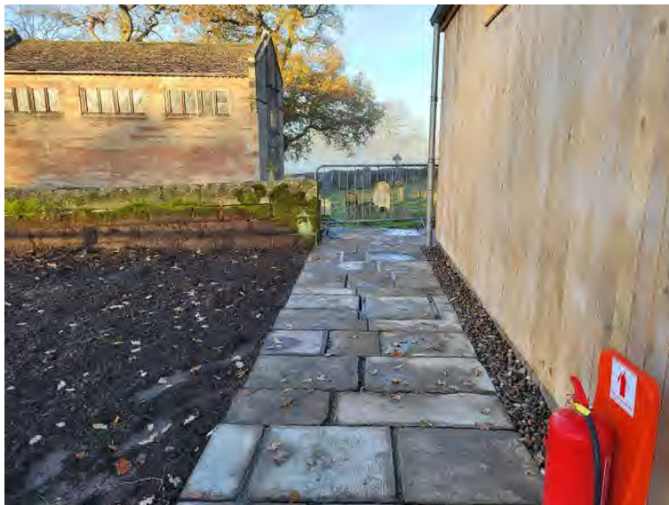
Figure 5: Landscaping - Stone Paving and Manhole Cover.
