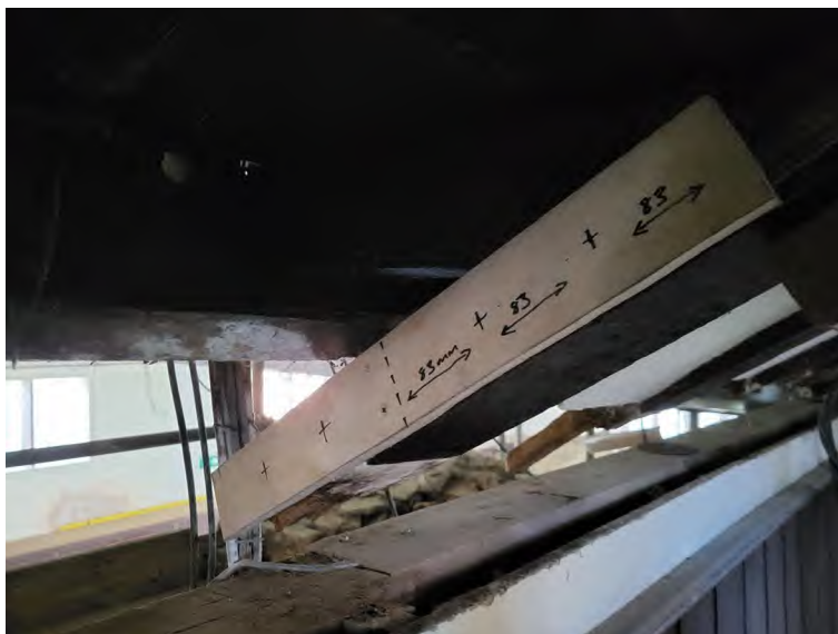
Figure 9: Timber Repair Works - Remedial Works to First Floor.
