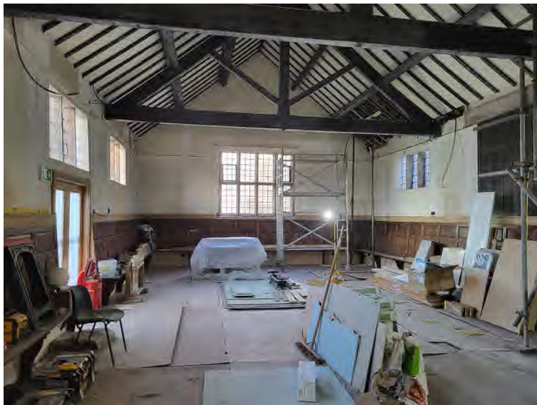
Figure 2: General View of Existing Hall.
