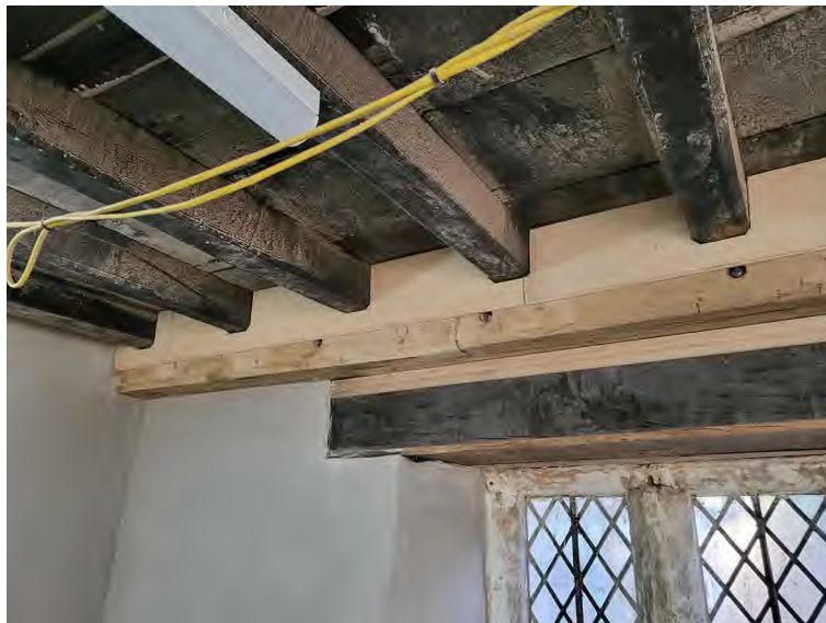
Figure 11: Existing Kitchen - Joinery to be Stained Dark.
