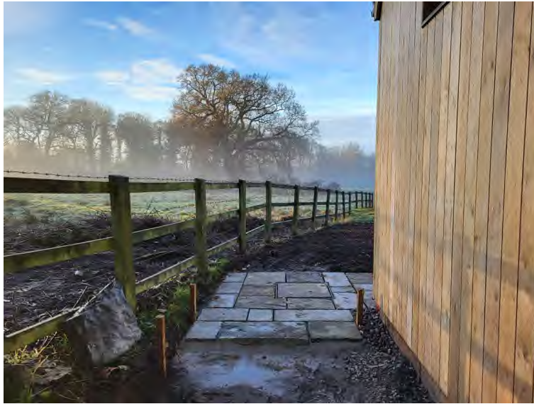
Figure 4: Landscaping - Stone Paving and Manhole Cover.
