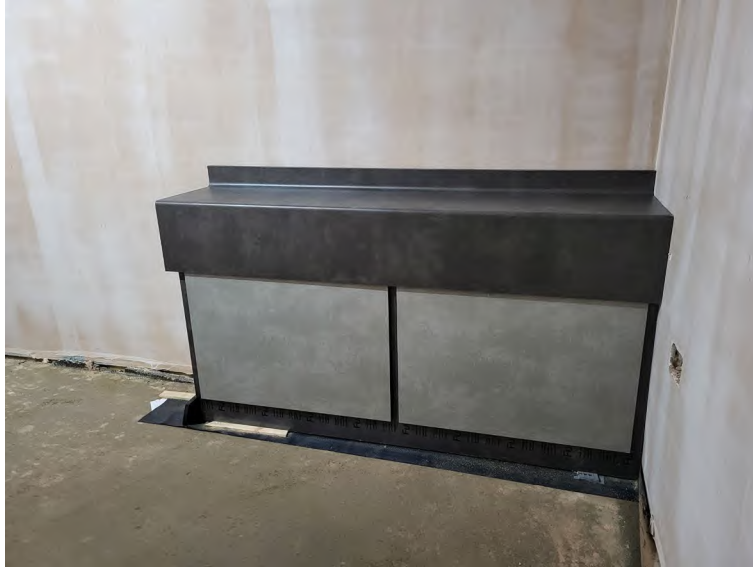
Figure 7: Female W.C. - Vanity Unit Installed.
