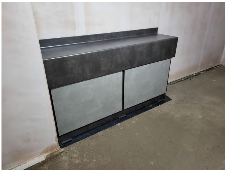
Figure 6: Male W.C. - Vanity Unit Installed.
