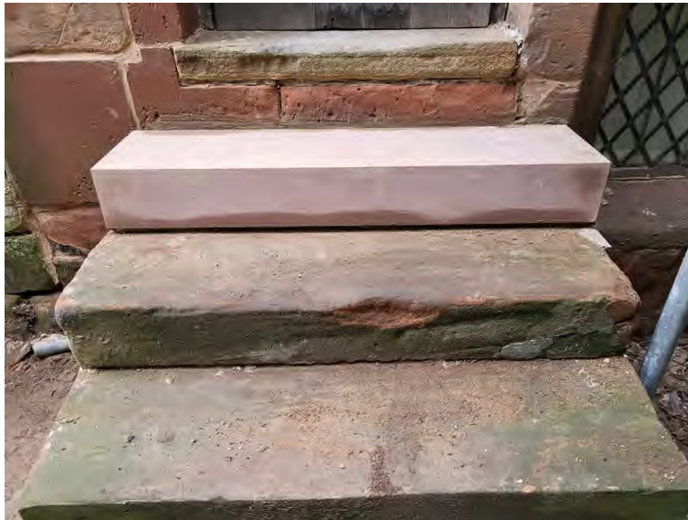
Figure 8: First Floor - New External Step.
