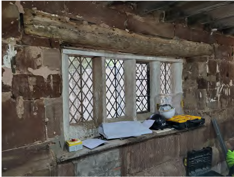
Figure 4: Existing Kitchen - Paint Removed.
