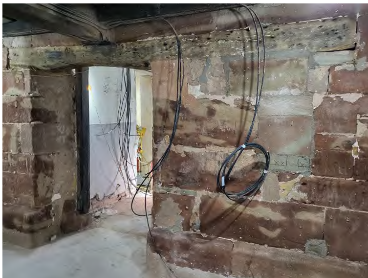
Figure 3: Existing Kitchen - Paint Removed.
